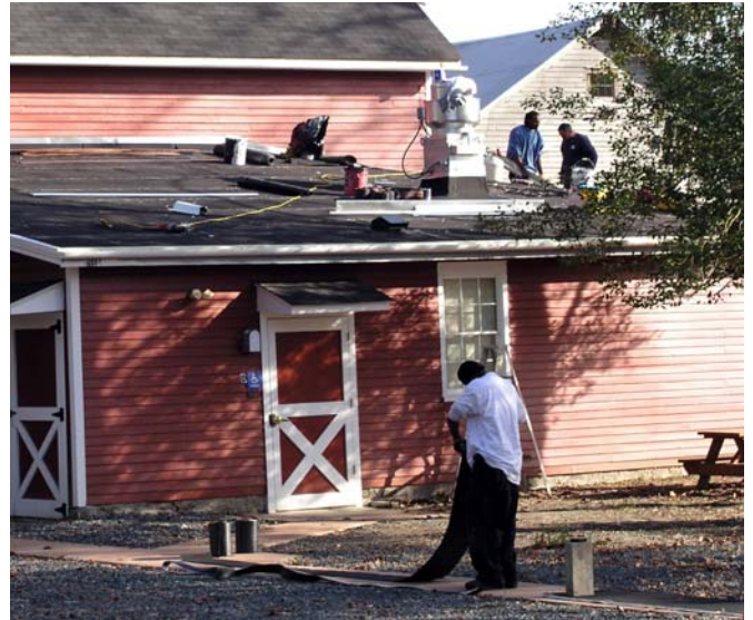
Workers installed a new roof on the barn, which houses the Commission's Science Office staff, during 2006. The building is located on the grounds of the historic Fenwick Manor.
