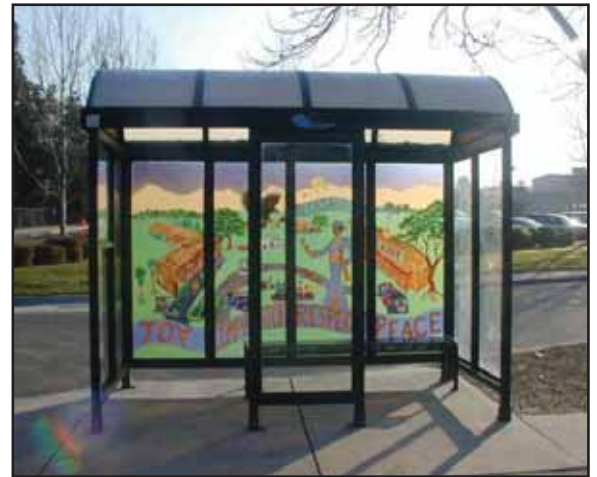
Bus shelters not only protect riders from the elements, they can be attractive parts of the streetscape that help to identify a community
