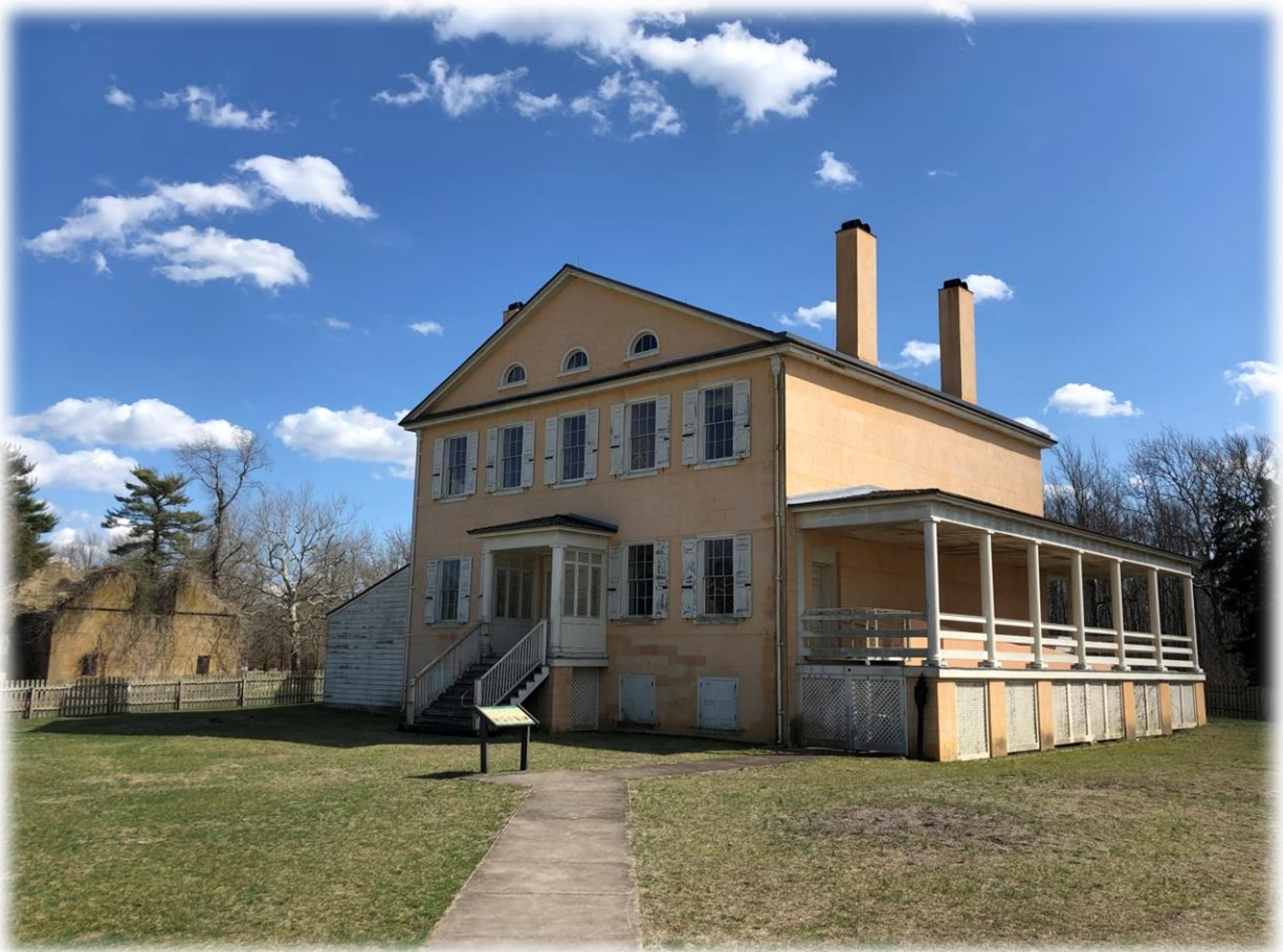
The Atsion Mansion in Wharton State Forest in March
